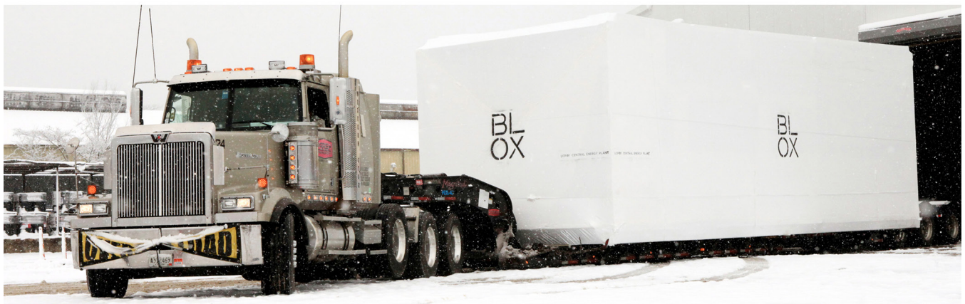
Figure 5. Top images: A single “manufactured chassis” of 15’x15’x60’ called “UBER” (first image) can host a series of programs for a healthcare facility (second image) that was built in 14 weeks (third image). Bottom image: A prefab module of 15’x15’x60’ manufactured by BLOX is transported to the job site (Images courtesy of BLOX).
