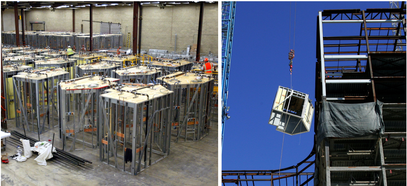
Figure 1. Left image: pre-fabrication of the bathroom modules in the offsite warehouse for the Miami Valley Hospital project designed by NBBJ Architects. Right image: A modular bathroom unit being elevated to its floor in the Miami Valley Hospital project designed by NBBJ Architects (Image courtesy of NBBJ architects).
