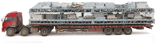
Figure 2. Top images: The 30-story hotel called T30 was built by Broad Group in China in only 15 days. Bottom image: each truck transports 2 pre-fabricated modules of the hotel. Bottom image: each module includes the floor and all the vertical elements that go above the floor (Image courtesy of Broad Group, China).
